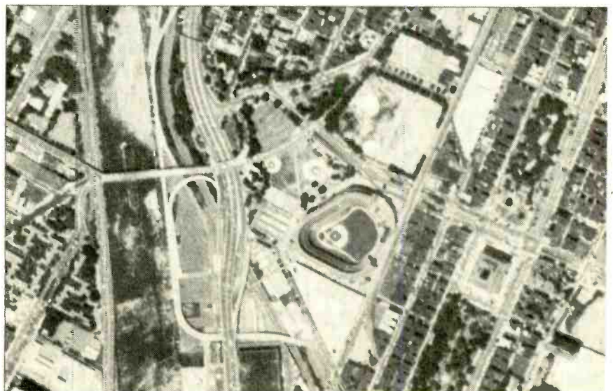
In this aerial photo of the Bronx, NY, you can see the "House that Ruth Built," along with the rest of the homes and roads in the area.
